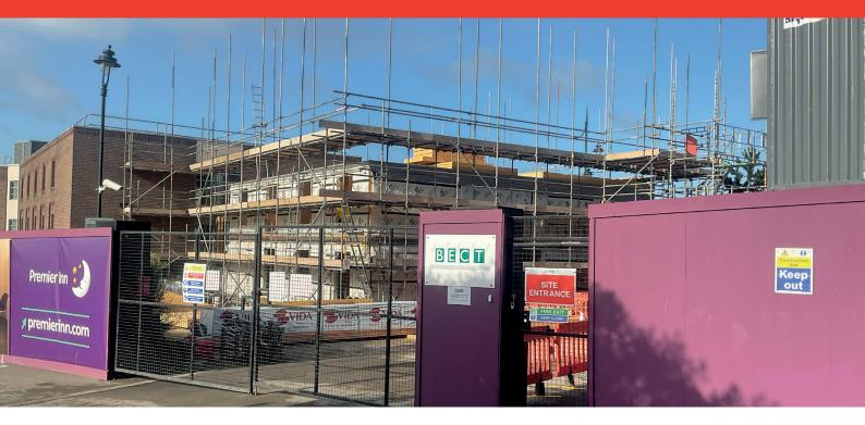
Crendon Timber Frame was appointed to design, supply, and install the full timber superstructure for a significant extension to the Premier Inn at Barry Island. The three-storey development on the north side of the existing hotel has added 21 new bedrooms and was delivered on behalf of the client, Whitbread Group Plc, for Bect Building Contractors Ltd.
