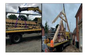
9. When offloading ensure you always have sight of your load. Always unload to the nearest hard standing/ground only. Never lift products onto the building/scaffold etc.
