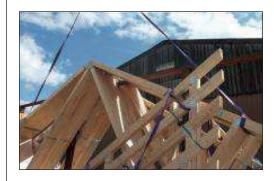
8. The driver will cut the individual 8mm blue rope attaching the pack to the centre bars. This must be carried out from a safe position using a telescopic cutting staff.
