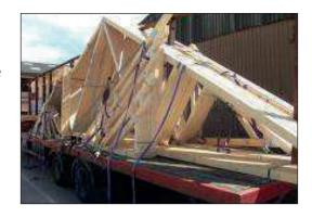
4. The manufacturer will supply truss packs secured to the trailer with 8mm blue rope. You should familiarise yourself with which rope attaches which pack to the centre bars.
