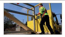
9. The driver will untie the 8mm blue rope then separate the 1st truss at the heel by hand or use of crowbar then replace the rope around the remaining trusses, repeating this process at the other end of the truss ensuring that, at all times, there is at least one rope securing the remaining trusses in the pack back to the centre bars.
