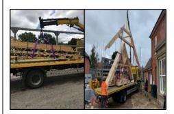
**8.** When offloading ensure you always have sight of your load. Always unload to the nearest hard standing/ground only. Never lift products onto the building/scaffold etc
