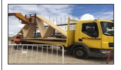
**6.** When instructed that the area is clear the FLT Operator shall remove the trusses from the lorry.
