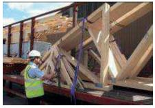
**3**. The manufacturer will supply truss packs secured to the trailer with 8mm blue rope. You should familiarise yourself with which rope attaches which pack to the centre bars.
