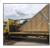
5. Safety Area Forked equipment will then lift the panel from the bed of the trailer. Given the weight and shape of panel it is essential that the danger area in front of the panel is kept clear of all personnel. NEVER stand in the danger area where the panel could potentially fall or swing. Do not allow any others to enter the danger area.
