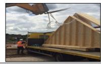
4. Lifting. The Lifting equipment will then take up the slack of the lift. On instruction from the site responsible person the driver will release the panel by cutting the blue rope. This must be carried out from a safe position using a telescopic cutting staff. The panels will have a short circular strap attached at one of the corners for guide use if required
