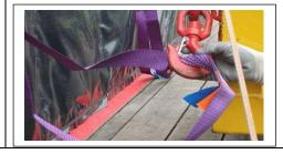
**3.** Slings. Drivers and site staff are not permitted to access lorry bed during unloading. Spandrel Panels will arrive preslung with appropriate 7:1 lifting slings. These slings are designed to be attached to crane hooks from ground level. Where Panels are delivered in sections always check supplier information for lifting and assembly details.
