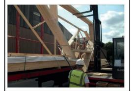
8. The forklift will then remove the truss pack from the trailer, position the apex of the pack onto the floor and reverse back slowly lowering the boom. Bearers can be used to support the underside of the pack. **9.** Once lowered the forklift will remove the forks and re-invert the truss pack at the apex. Once fully supported the truss pack can then be moved to its location.
