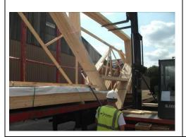
**8.** The forklift will then remove the truss pack from the trailer, position the apex of the pack onto the floor and reverse back slowly lowering the boom. Bearers can be used to support the underside of the pack.
