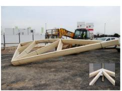
**9.** Once lowered the forklift will remove the forks and re-invert the truss pack at the apex. Once fully supported the truss pack can then be moved to its location.
